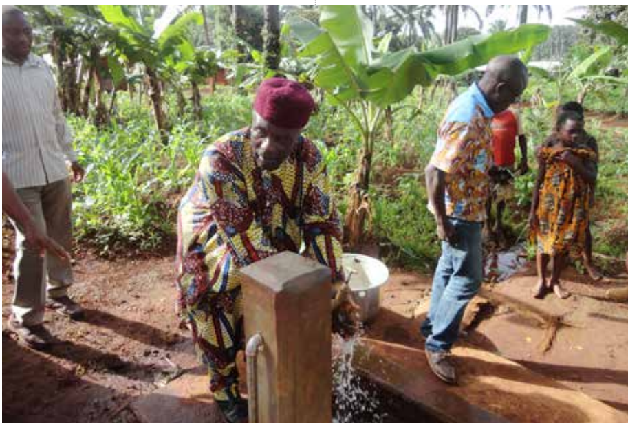
Reception of water project in Bangolan by 2 nd Deputy Mayor of Babessi
